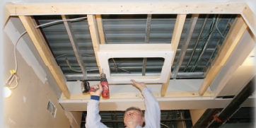
2. Mount Seamless™ surround with drywall screws.
