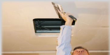
5. Tape and apply drywall compound.
